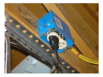
Exposed/loose/hanging wires noted at the rear wall of the garage. This is a safety concern if used where it could be subject to physical damage or accidental human contact. Wires were not 'live' at the time of inspection, although inspector cannot determine if wires could be made live by an unidentified circuit breaker or switch. Client should consult with a qualified electrician for removal or proper termination as needed to avoid shock hazard.
